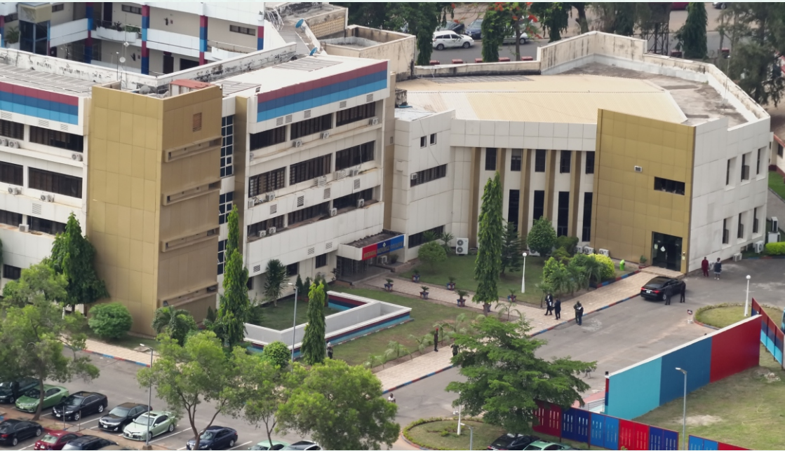
National Defence College Complex Abuja
