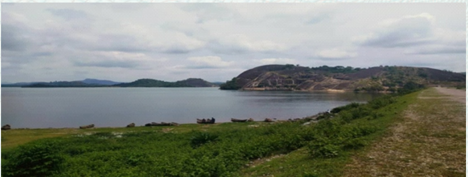
Usman Dam (40km from the College)
